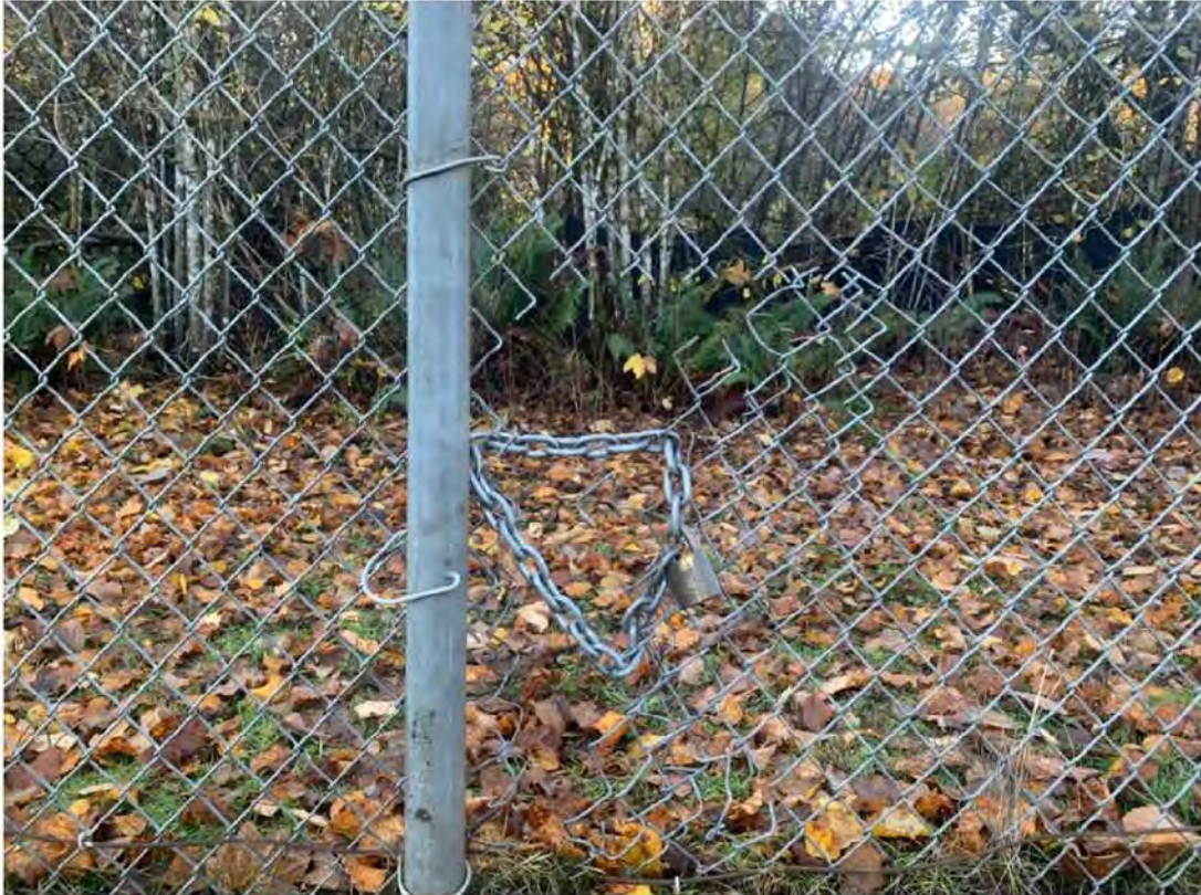
A chain link fence with a lockDescription automatically generated
