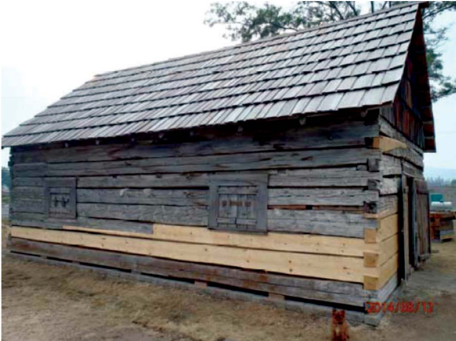
Figure 25. North Elevation of Skolaskin's Church, Phase II Project Stabilization.
