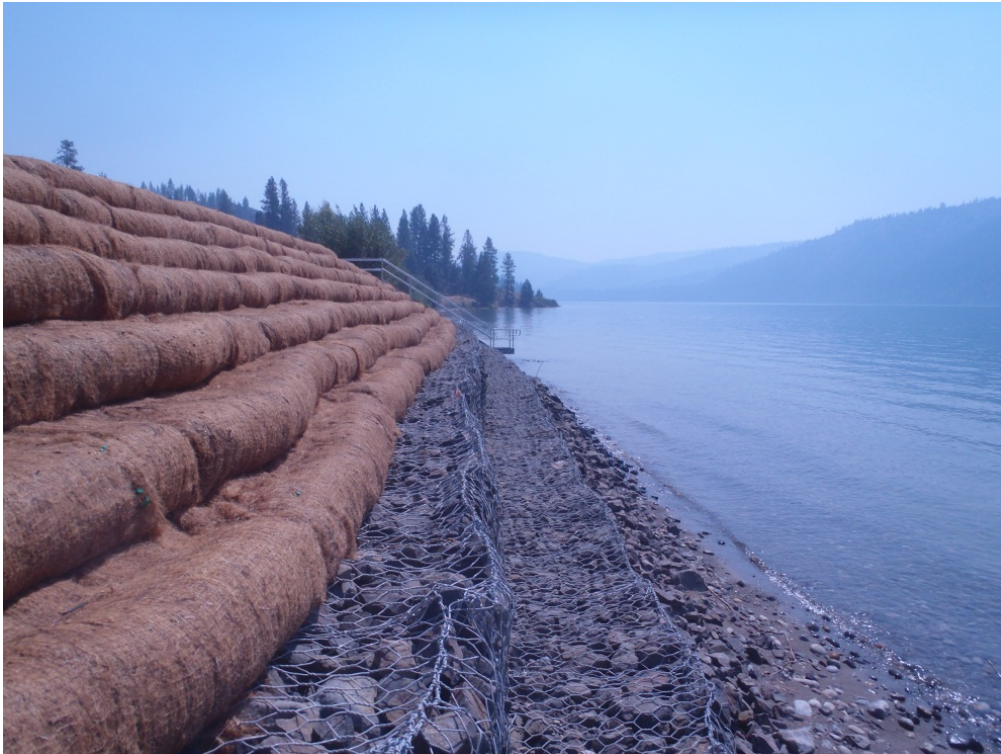
Figure 22. Stabilization on Spokane Arm at Substantial Completion, July 2013.
