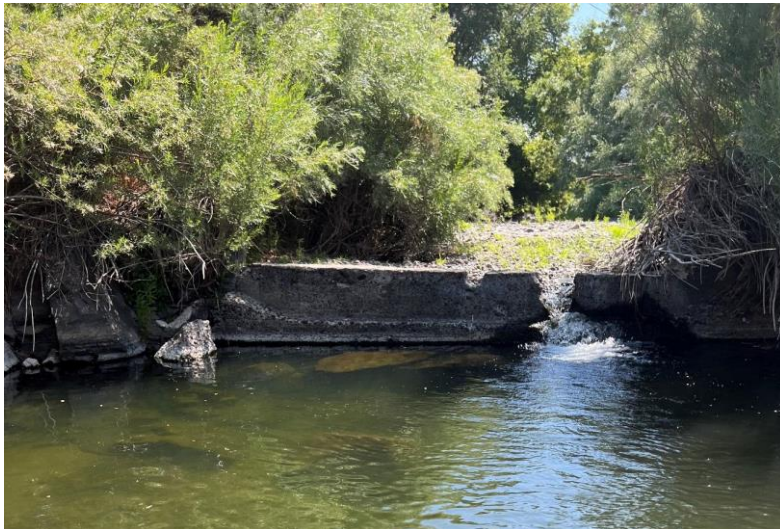
Figure 2. Current conditions at Peterson Dam.
