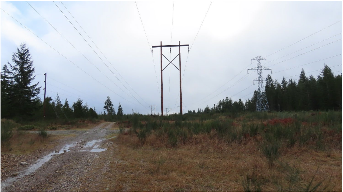
Figure D-1: Existing Two-Pole Wood Structure
