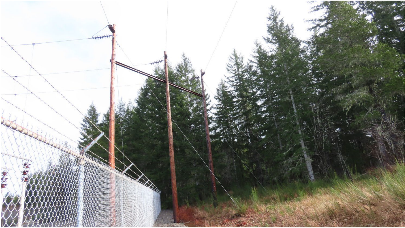
Figure D-2: Existing Three-Pole Wood Structure
