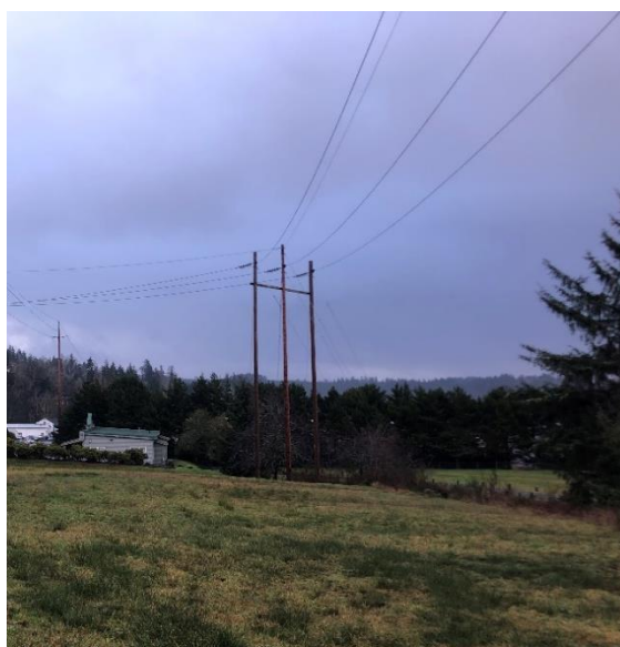
Figure 2-1. Existing Two- and Three-Pole Wood Structures
