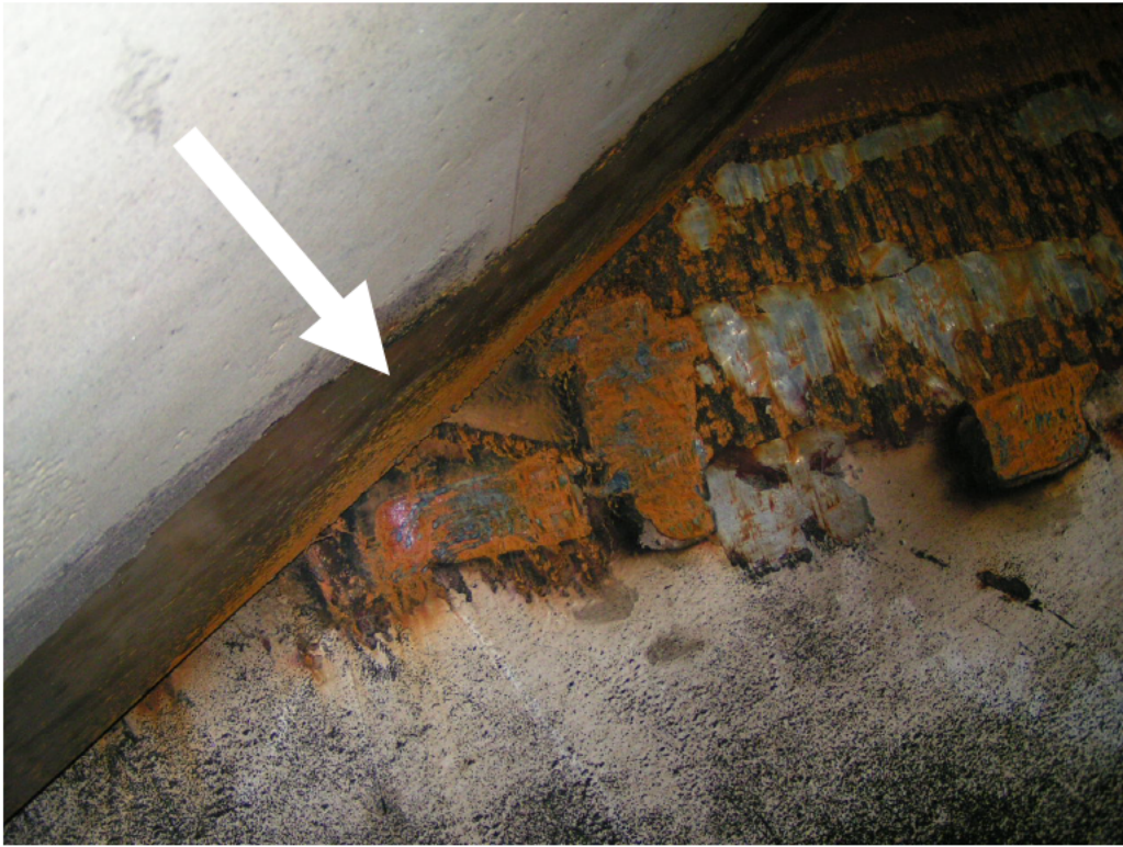
Picture 4: Typical Turbine Blade Cavitation Damage at Blade End
