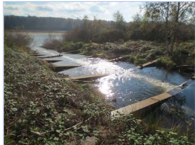
Photo 2-2: Gibbons Creek fish ladder looking south.
