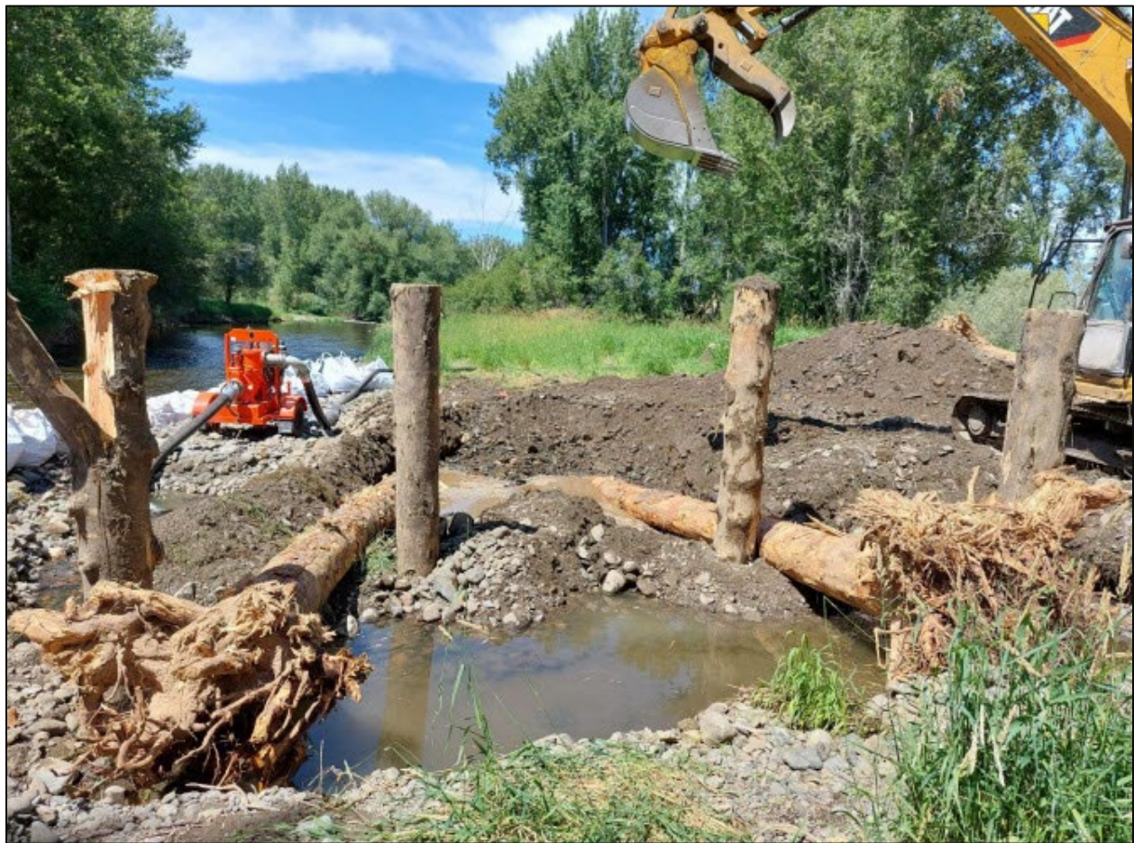
Figure 20: 2022069(Lostine Side Channel)LWD Install
