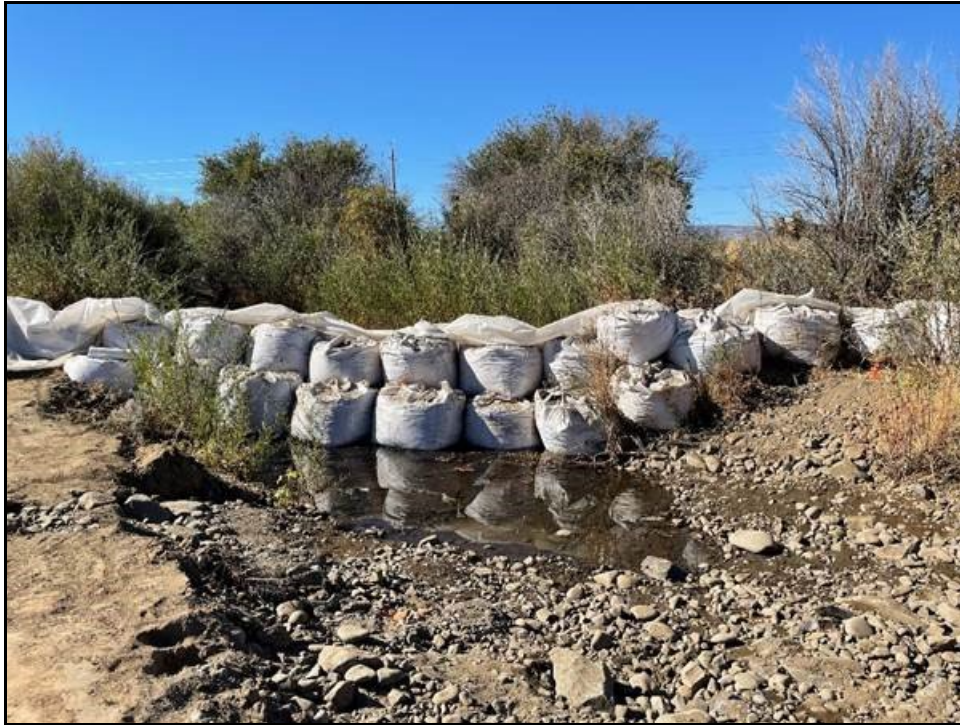
2022073(Simcoe Creek) Cofferd Dams
