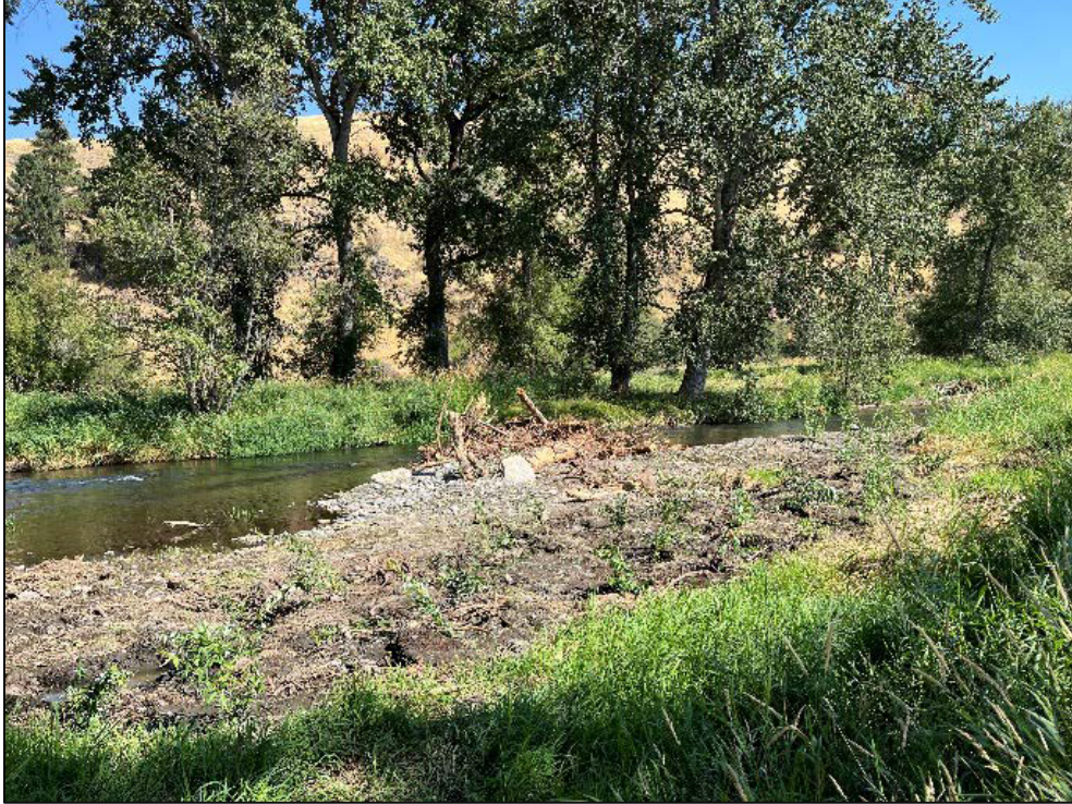
Figure 15: 2022056 Wilson Haun Apex Structure
