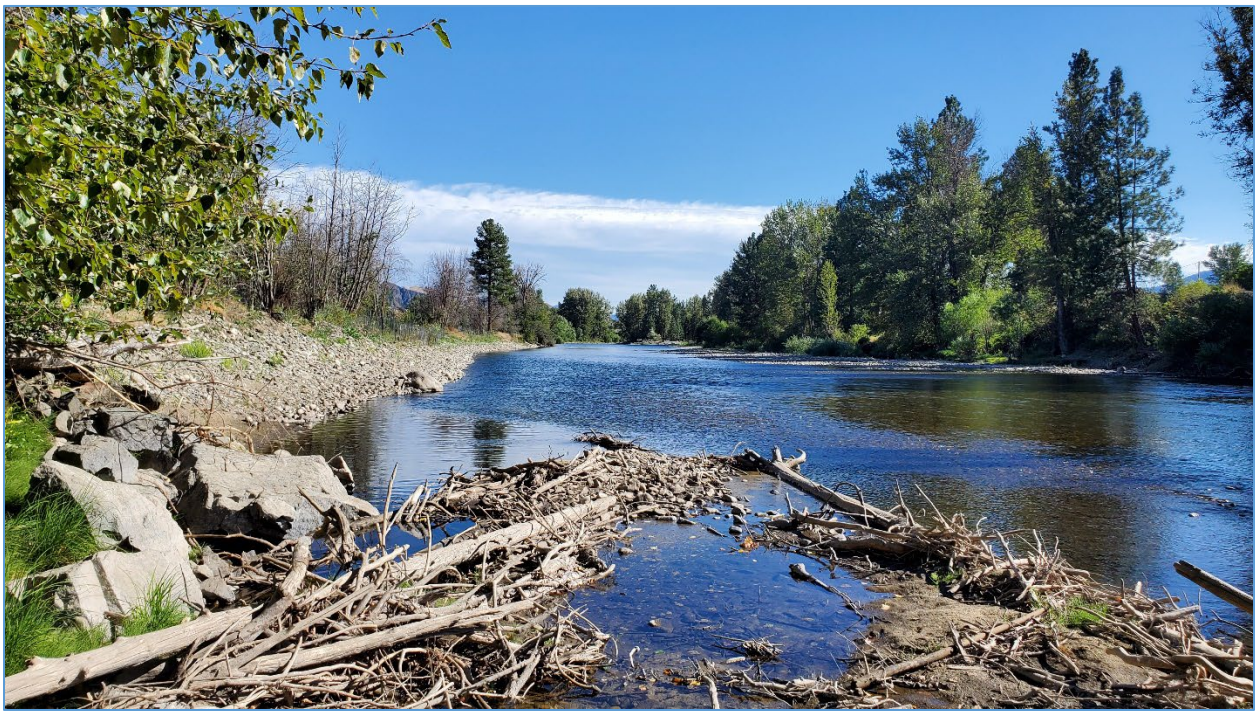
Figure 18: 2022088(Barkley Bear) Levee Removal Area
