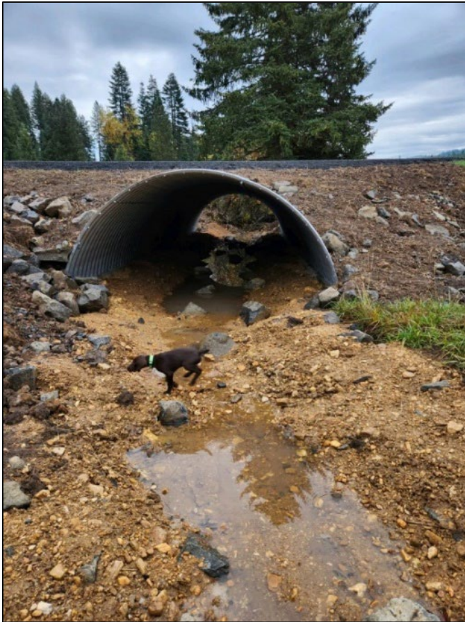
Figure 19: 2022042(Crocker Creek)Culvert Replacement, before and after
