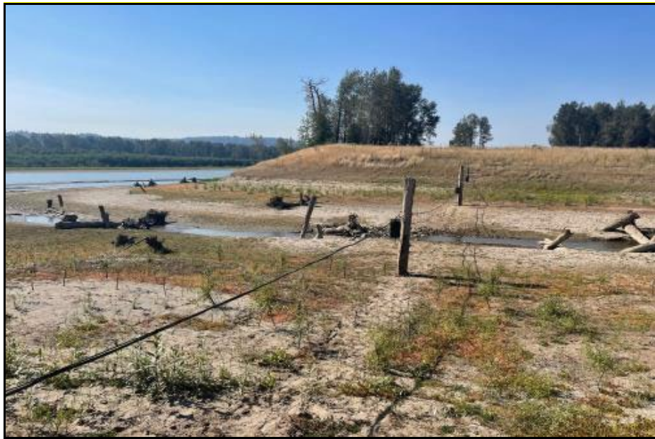
Figure 10: 2022016(Stiegerwald)Pit Array Installation
