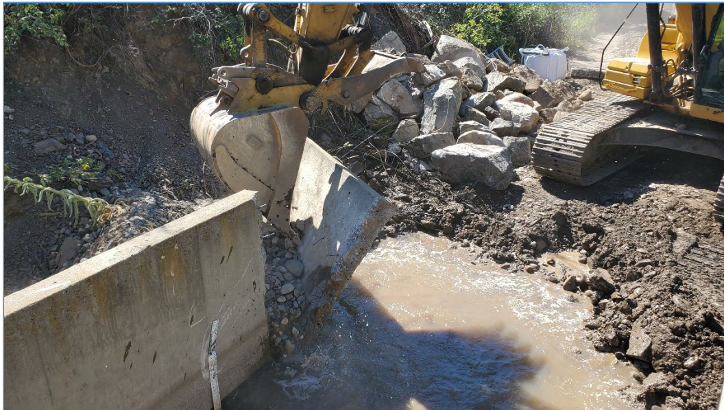
Figure 16: 2022088(Barkley Bear) Headgate Removal
