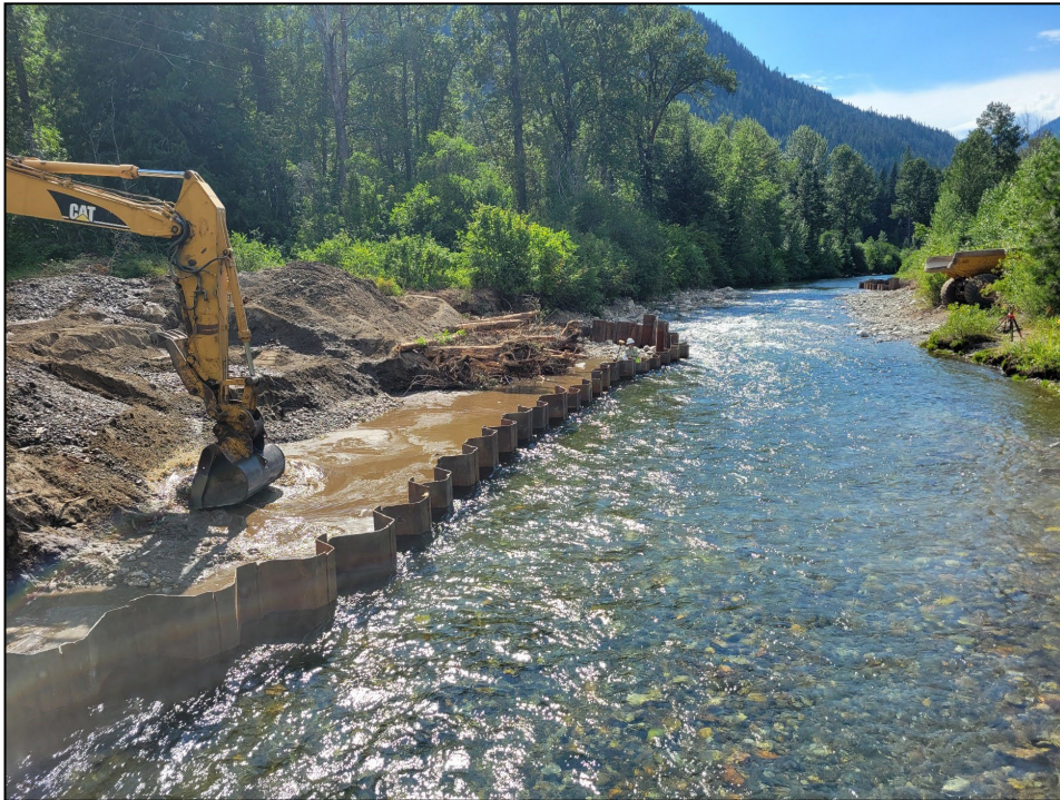
Figure 13: 2022023(M. Oxbow)ELJ Install
