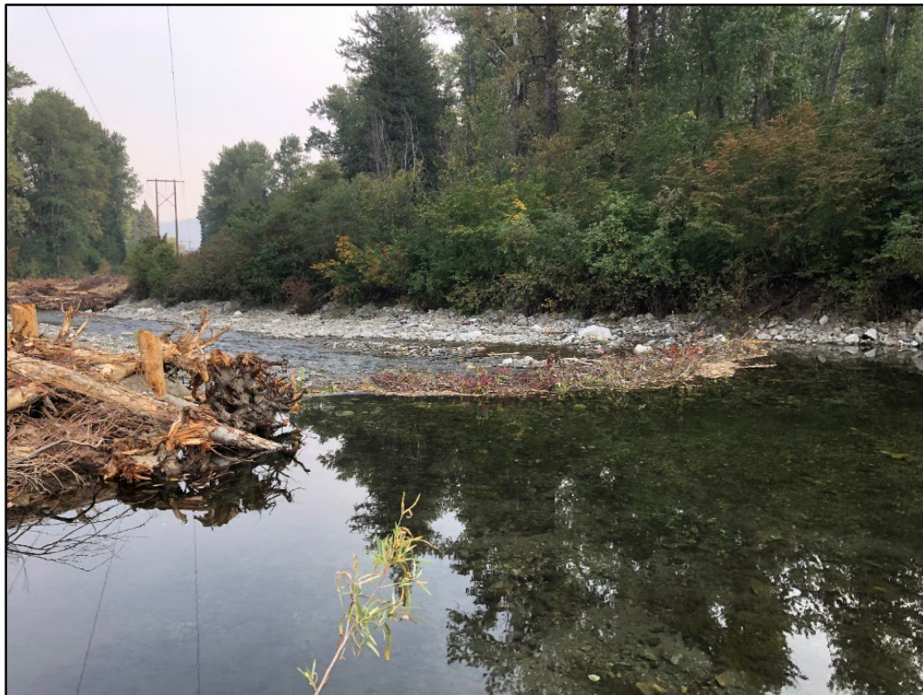
Figure 11: Top of roughend channel (beaver activity post construction)
