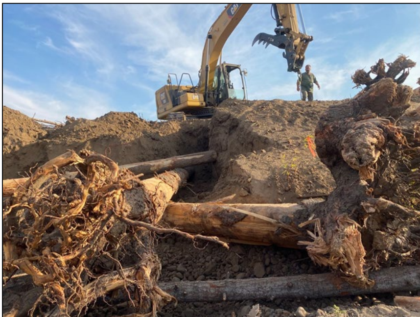
2022073(Simcoe Creek) Excavation
