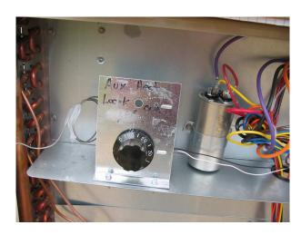
Ohmmeter between the control terminals, and turn the adjustment dial until the circuit is closed (resistance on ohmmeter goes from infinite to 0 or near 0). If the circuitry does not make/break right around 32° F, the control will have to be exchanged for another control.
