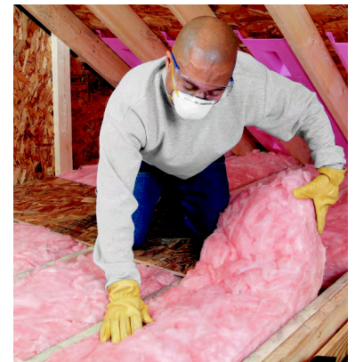
Batt insulation installation
