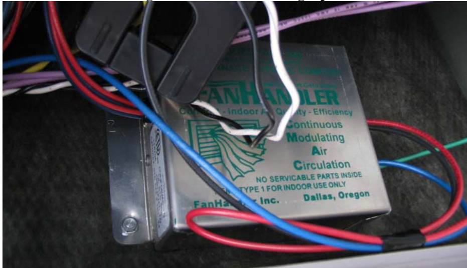
Figure 4. Fan Handler Single-phase VSD
