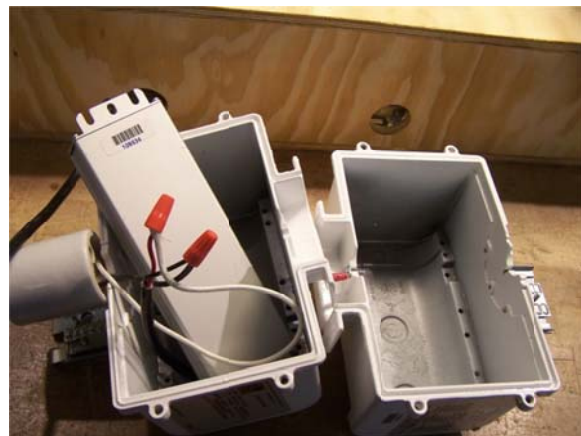
Figure 23: External LED drivers for mogul base replacement lamps mounted in luminaire ballast enclosure (HB1 on left, HB6 on right)
