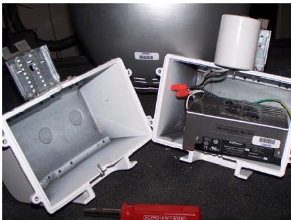
Figure 23: External LED drivers for mogul base replacement lamps mounted in luminaire ballast enclosure (HB1 on left, HB6 on right)
