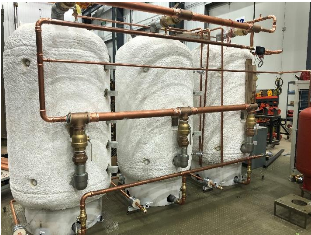
Figure 2. Storage tanks and piping during initial skid assembly. Photo credit: Steffes.
