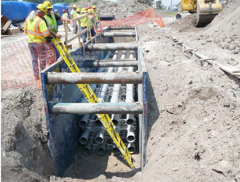
FIGURE 2-8 UNDERGROUND CABLE CONSTRUCTION ROW WITH SINGLE CABLE OPEN TRENCH
