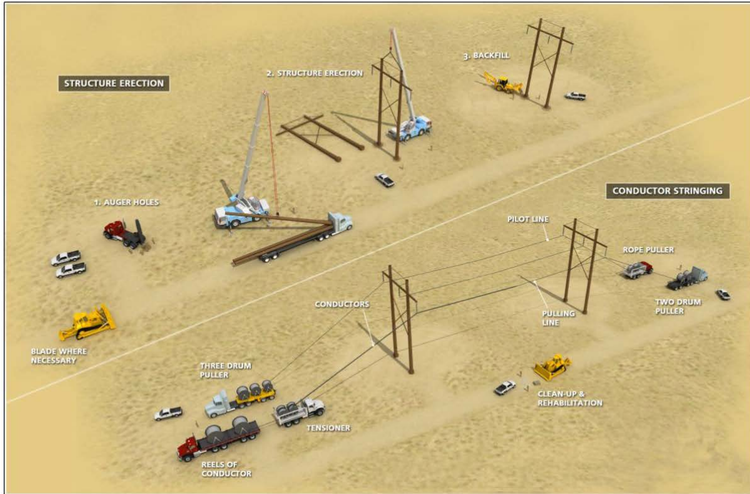
FIGURE 2-6 TYPICAL STRUCTURE ASSEMBLY AND WIRE INSTALLATION ACTIVITIES
