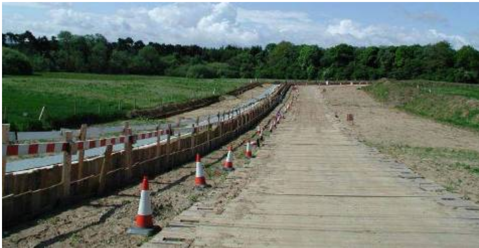
FIGURE 2-8 UNDERGROUND CABLE CONSTRUCTION ROW WITH SINGLE CABLE OPEN TRENCH
