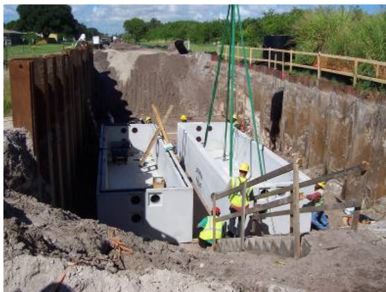
FIGURE 2-9 TYPICAL UNDERGROUND VAULT INSTALLATION (EPRI 2008)
