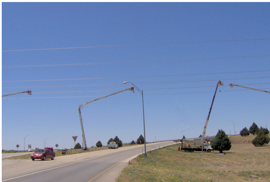
FIGURE 4.7-1 HIGHWAY CONSTRUCTION STRINGING ACTIVITIES
