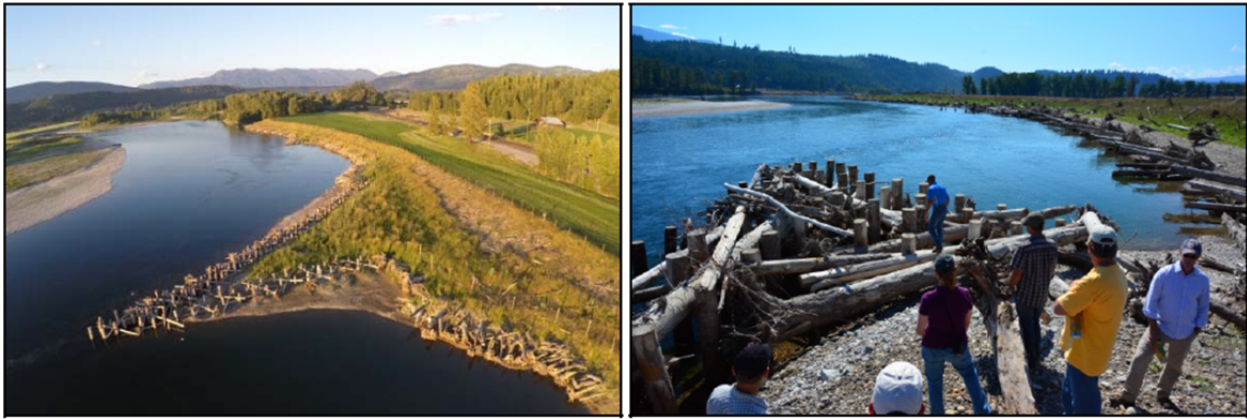
Figure 5. Examples of large bank structures in the Kootenai River
