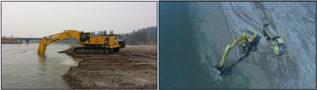
Figure 6. Pool excavation actions in the Kootenai River
