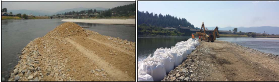
Figure 9 Examples of temporary river access road construction
