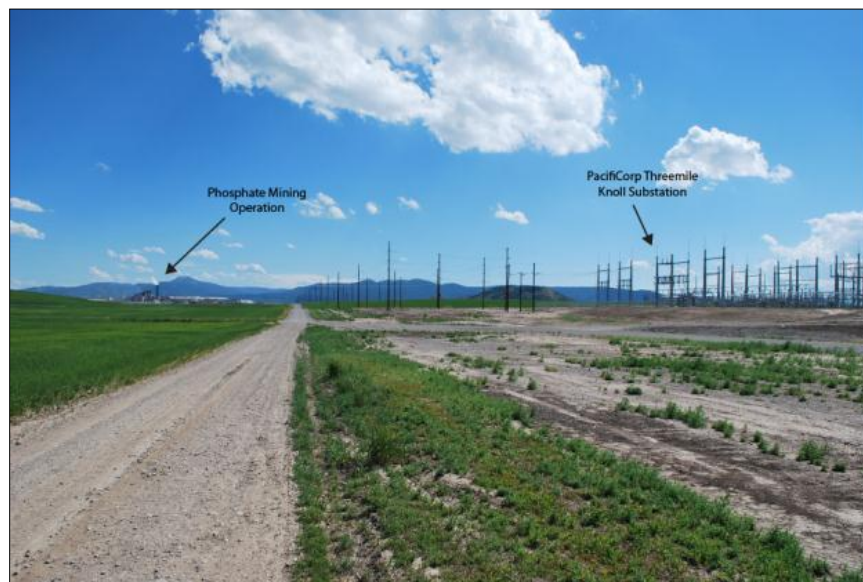
Figure 3-1. Photo 1—Vicinity of the Proposed Hooper Springs Substation
