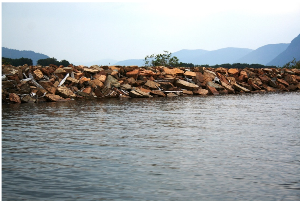
Figure B-7: Example of existing riprap breakwater at Area 3.
