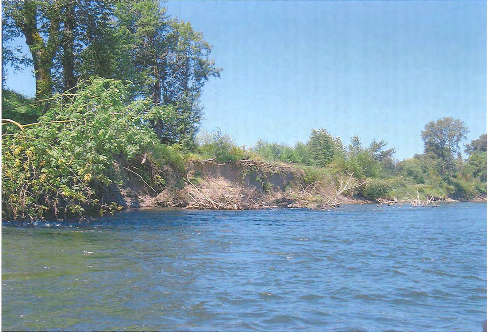
Figure 16 Bank Erosion Near River Mile 62
