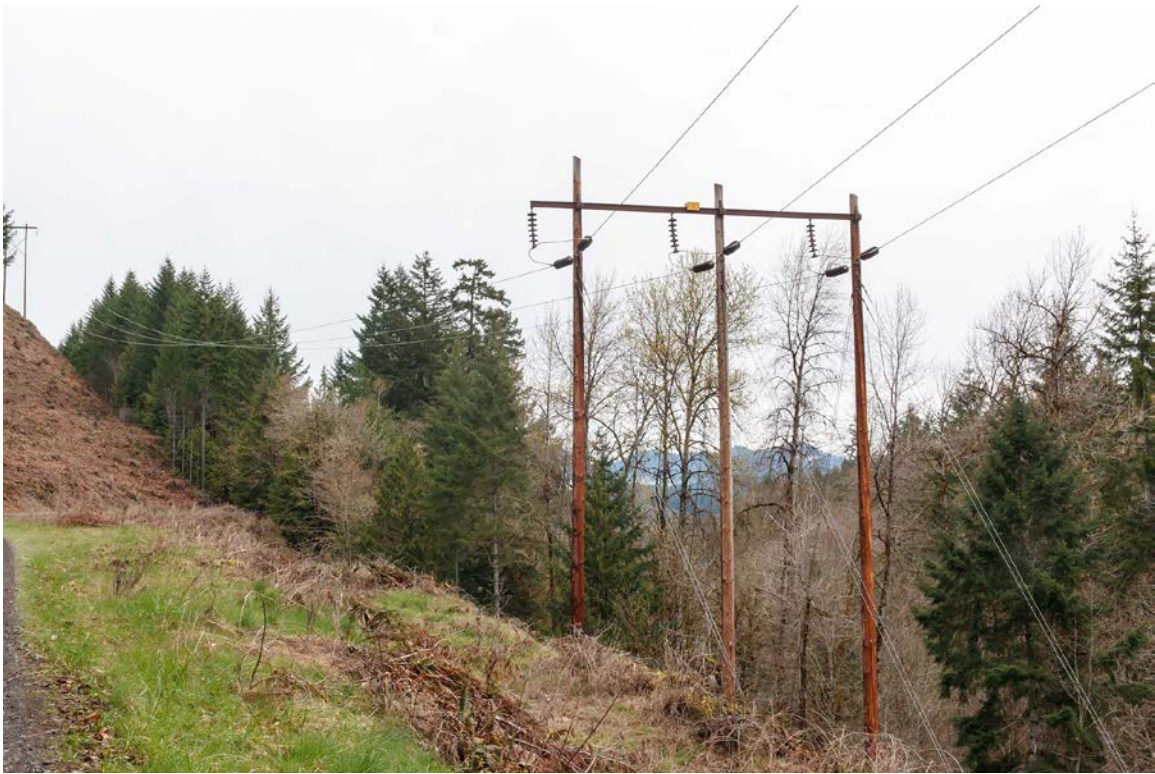
Figure 2-3. Existing Three-Pole Wood Structure (Line Mile Three)
