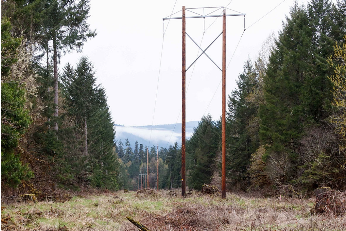
Figure 2-2. Existing Two-Pole Wood Structure (Line Mile Three)
