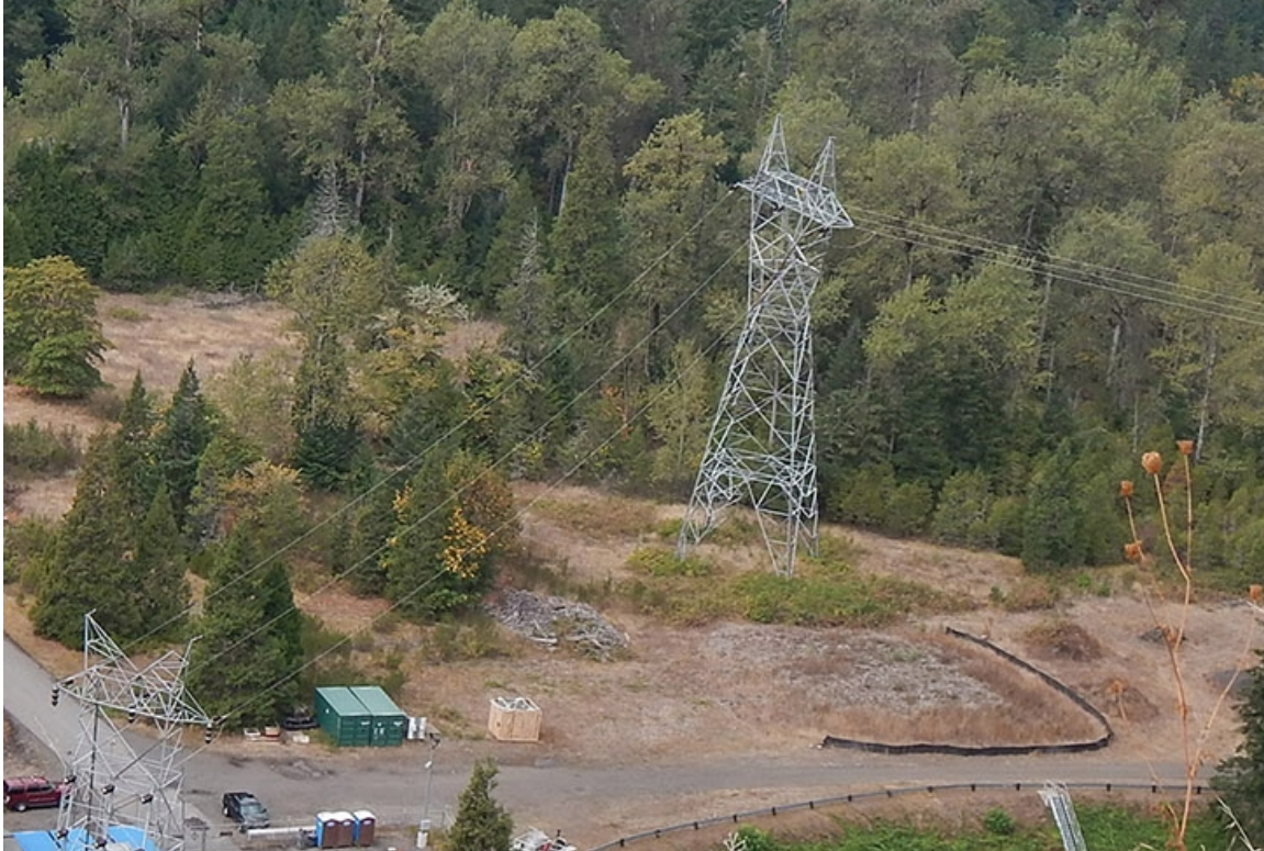
Figure 2-1. Existing Steel-Lattice Tower (Line Mile One)
