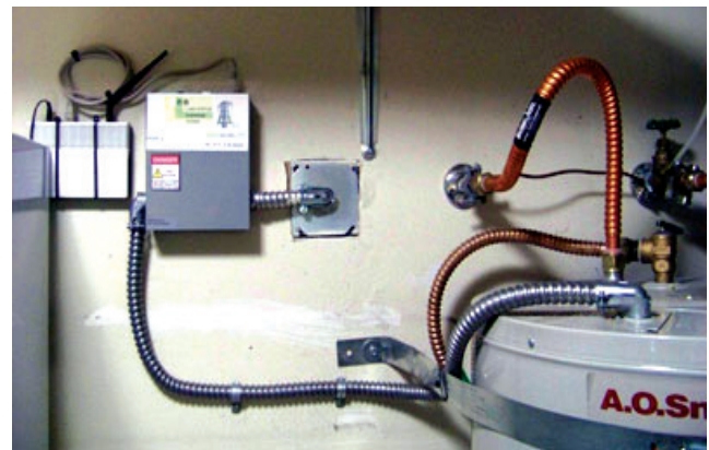
Demand response controllers on residential equipment such as water heaters can help grid managers keep the power system in balance.
